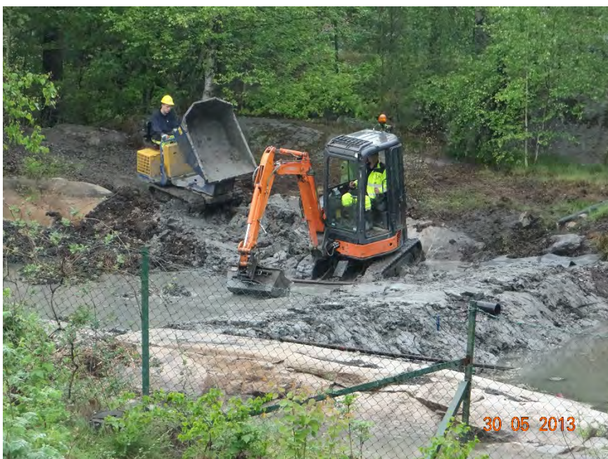
Gravemaskiner lager demning.
