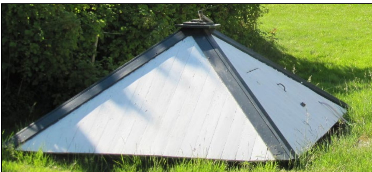
Figur 23: Pyramideformet brønnhus, ID 271086-2.
